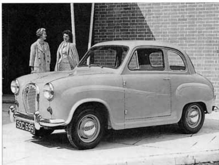
same body as the A30, it could be distinguished by its larger rear window, painted grille (the A30's was chromed) and remote control gearbox with more evenly spaced ratios. To the driver the improvement was immediately apparent, the A35 having a top speed of 75mph, some 10mph more than that of the earlier model.
